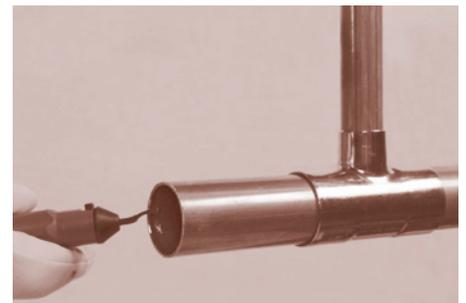
Figure 6. Fluxing: Tube
