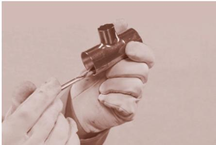
**Figure 8. Removing Excess Flux**
