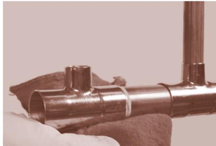
**Figure 9. Soldering**
